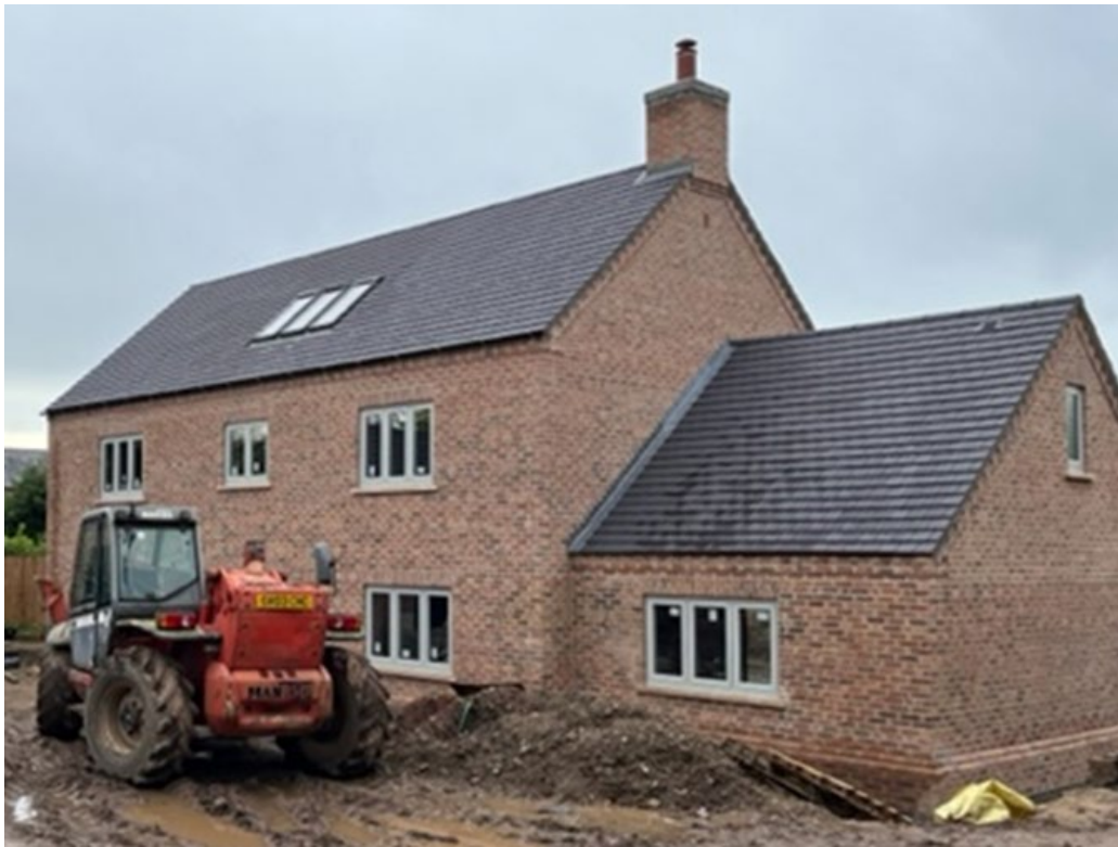
Photograph of the rear/west side elevation as built on site:
